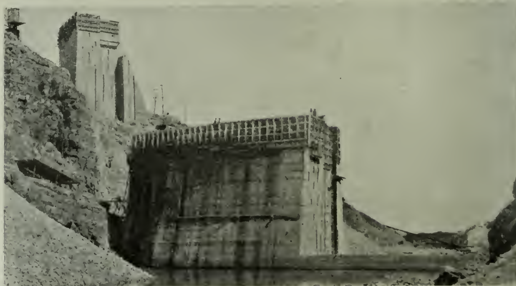
HARTEBEESTPOORT DAM, LOOKING DOWNSTREAM (February 2, 1922).
